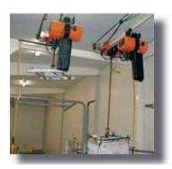
Example of special low headroom Hitachi hoist and trolley in food manufactuing plant
